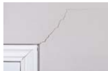
Cracking due to Shrinkage/Drying Out
