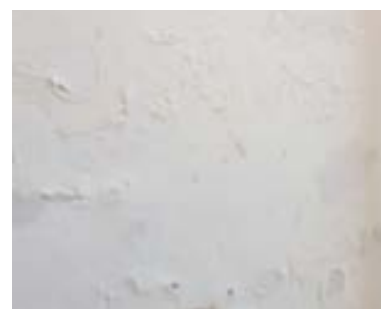
Efflorescence on Brickwork
